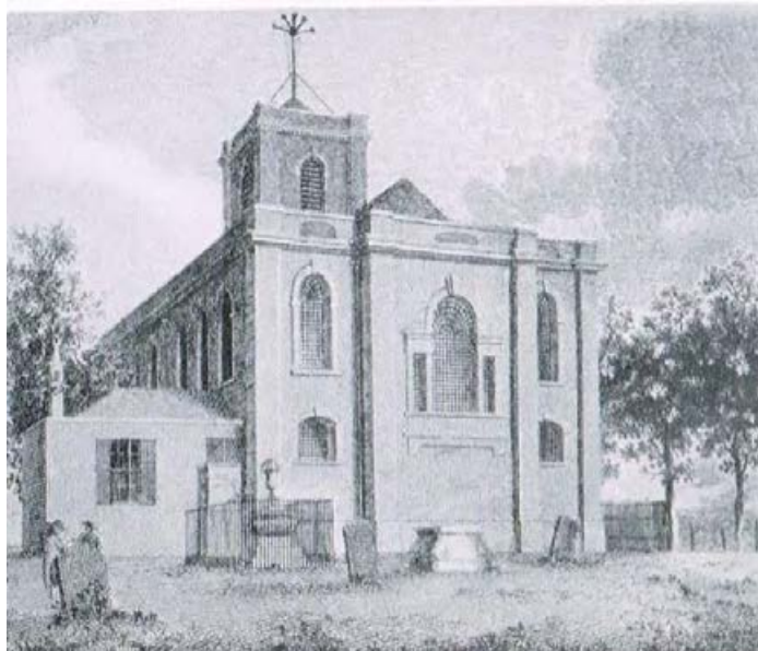
Woolwich Parish Church showing the Revd Mr Gamble's experimental radiated telegraph on its tower: correspondence was made with a similar apparatus on Shooters Hill, near the shutter telegraph station.
